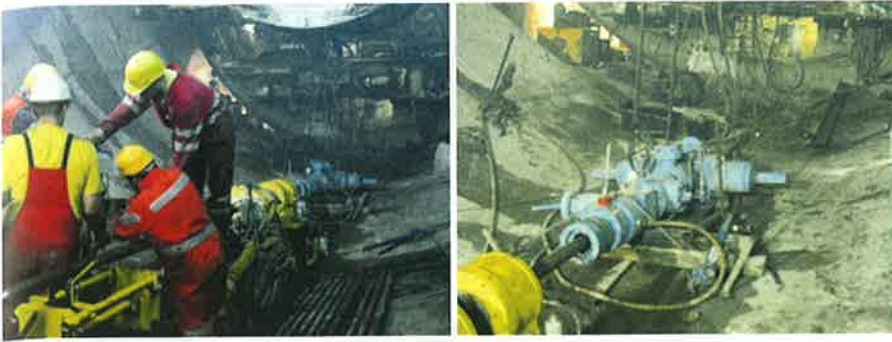
Fig. 9. Counter flush drilling with Diamec, Gotthard Base Tunnel, Amsteg contract
